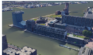
2 St. Jobshaven Terminal
